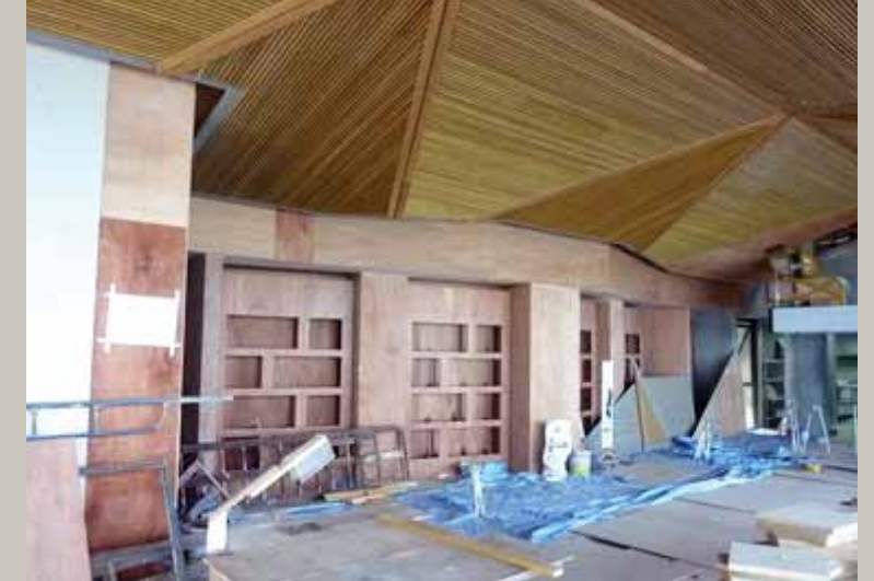
ABOVE | LATTICE CEILING
